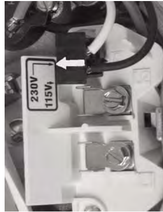
Figure 5A -Voltage Change Plug Set for 230 Volts.
