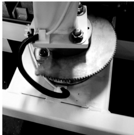
Figure 4: The cable, as it should appear to be under the Housing cover.
